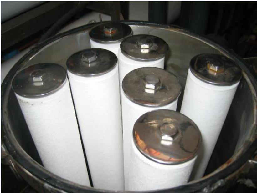
Changed New Cartridge Filter 0.5 \mu\text{m} of RO Unit
