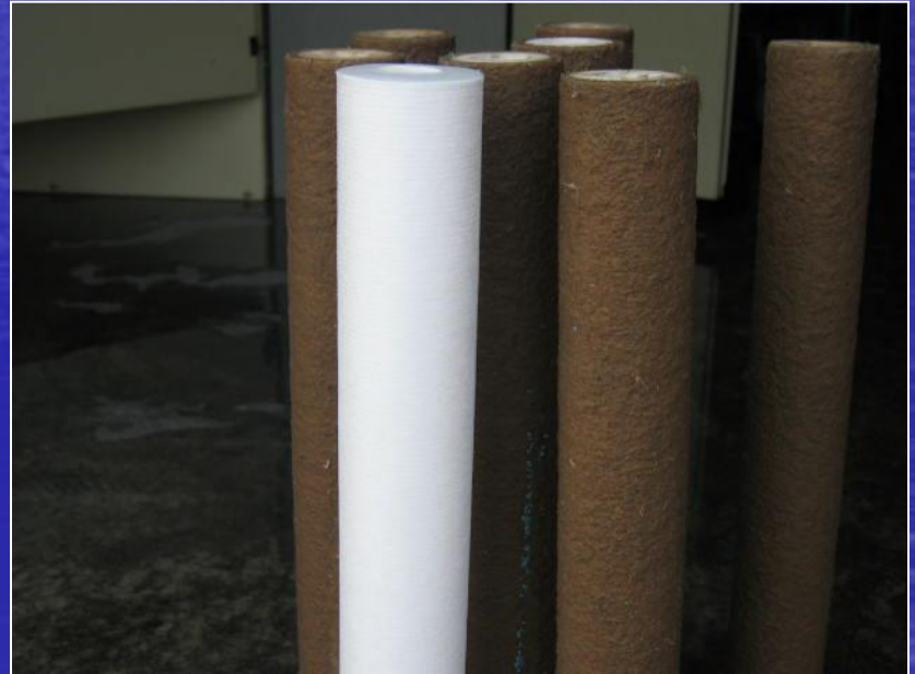
Changed New Cartridge Filter 0.5 \mu\text{m} of RO Unit
